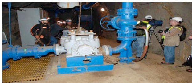
Newly installed 700 hp pump at the 2450 joins another one on that level
